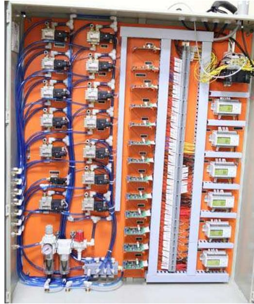
**Figure 2:** Electro-Pneumatic Control System
